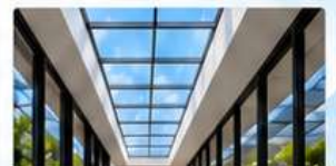
Commercial Skylight 📍 Bengaluru, KA
